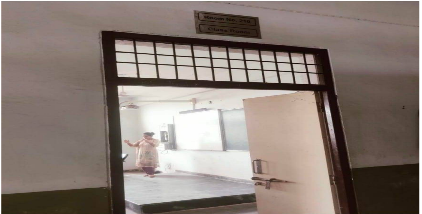
Class room with proper lights and ventilation :
